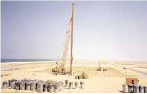
Above, the Port-Saïd soil consolidation site carried out by the use of prefabricated drains combined with an overburden consisting of temporary fill.
