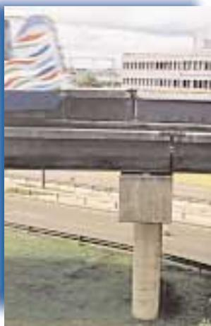
girder with two 82 m long cantilever spans. The structure is supported on bearings on
