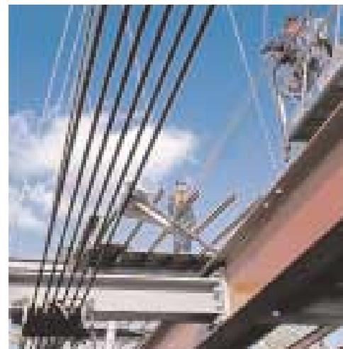
The deck was placed by incremental launching of the segments using a tensioned strands system between the banks of the Cher and pads with greased combs.
