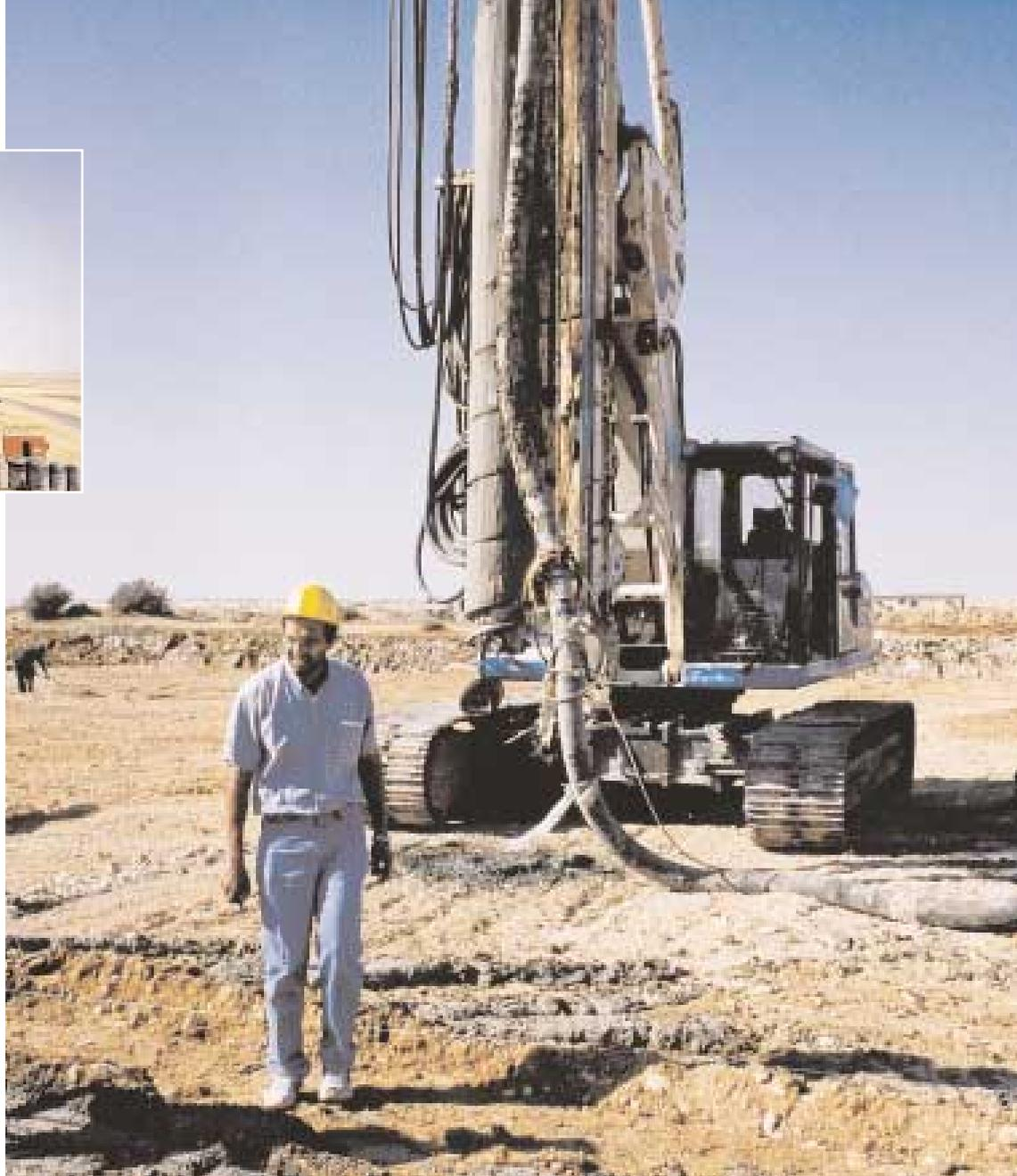
Menard Soltraitement used the controlled modulus columns (CMC) technique for the Suez site.
