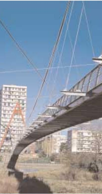
The Cher footbridge is a lightweight braced triangular shaped structure, derived from the footbridge constructed by the French engineer, Mr. Le Ricolais.
