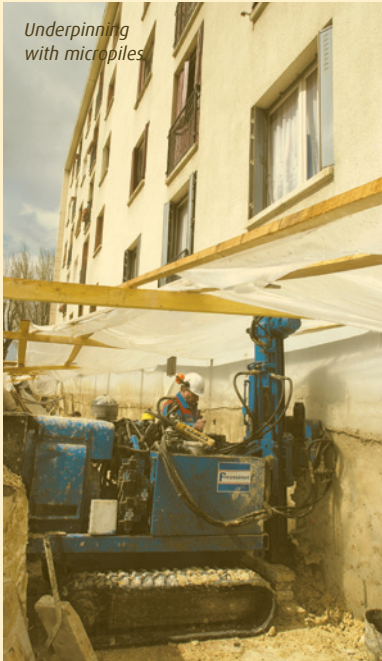
Underpinning with Fondapieux
