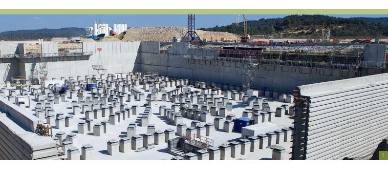
The composition of the elastomeric mixture determines the damping capacity of the ISOSISM® HDRB isolator.
