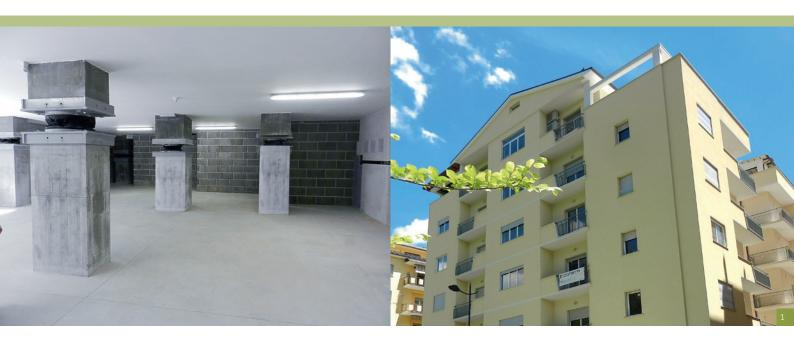
The type of PS isolator chosen depends on the nature of the structure to be isolated, the permitted displacement and the space available.
