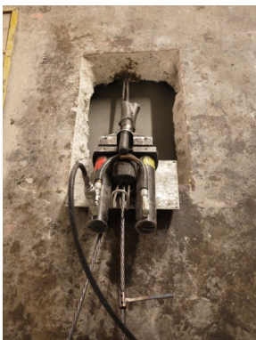
Tensioning operations
