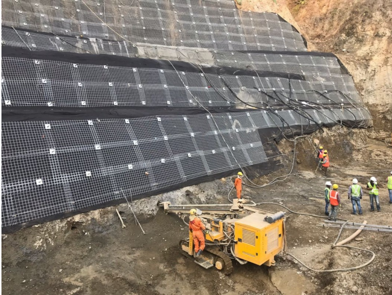
Soil nailing works
