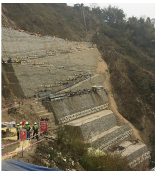
General view at half height progress
